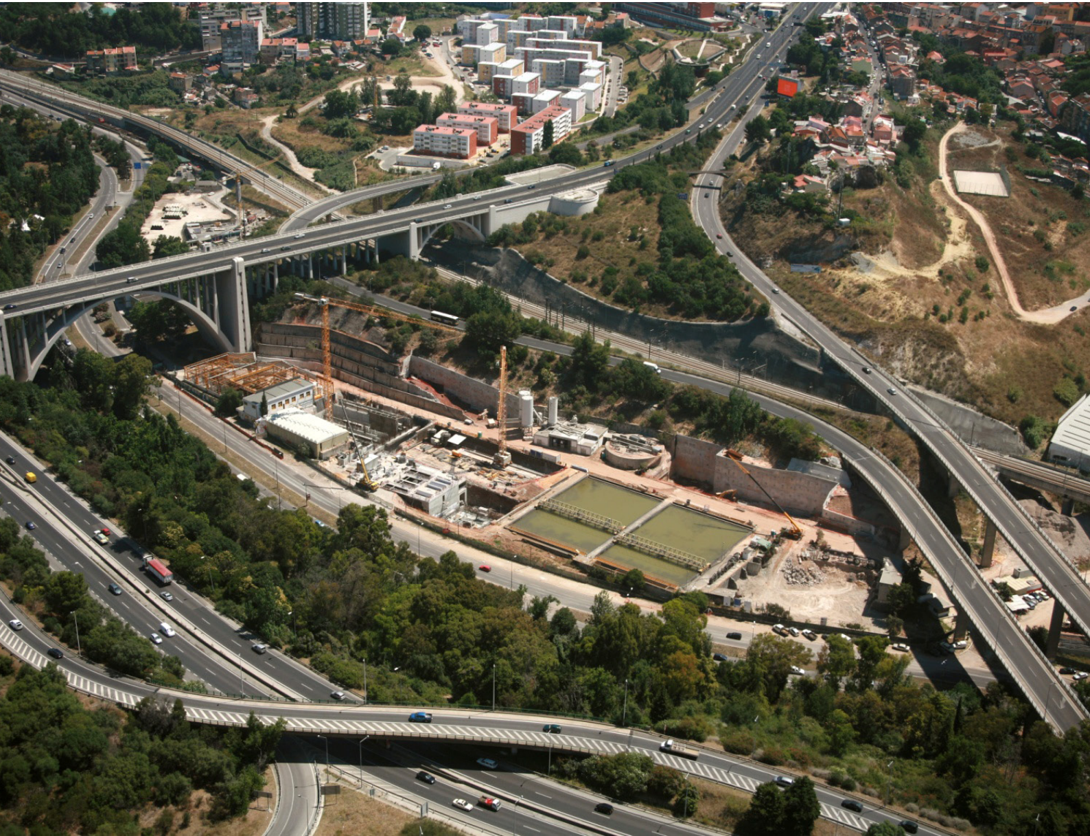
Aerial view of the site, before the intervention.
