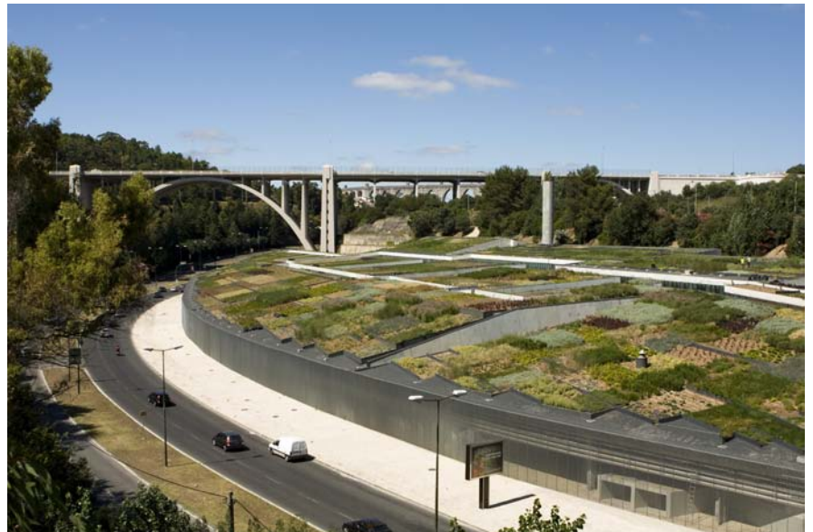
General views of the intervention site.
